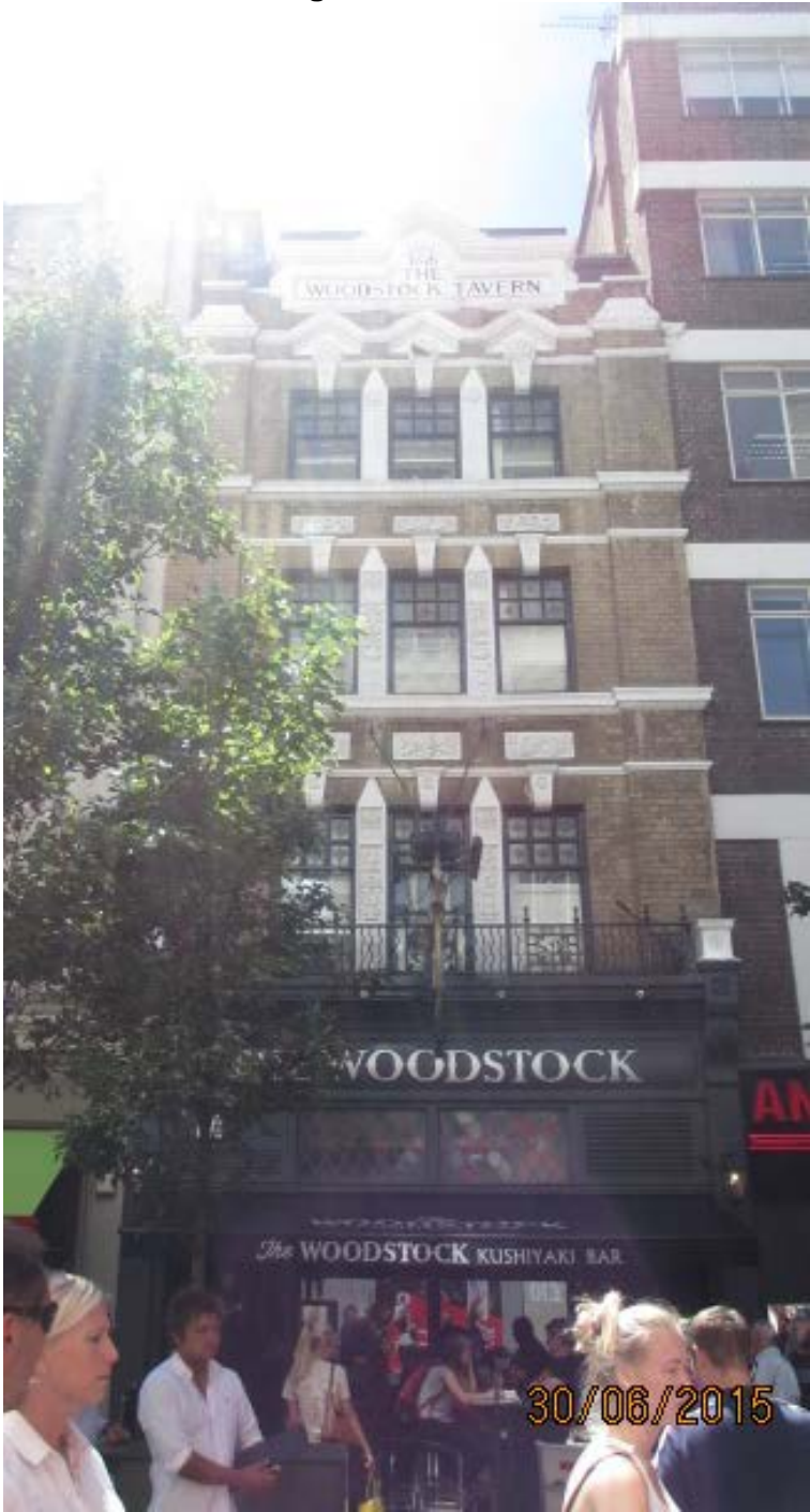
Photograph 1. Front elevation of building
